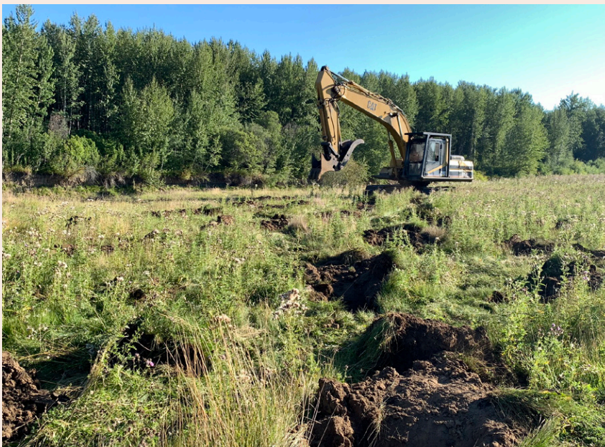
Site Preparation at Swan River First Nation
