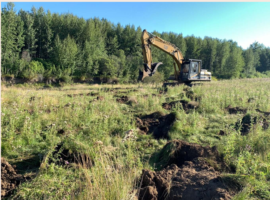
Site Preparation at Swan River First Nation
