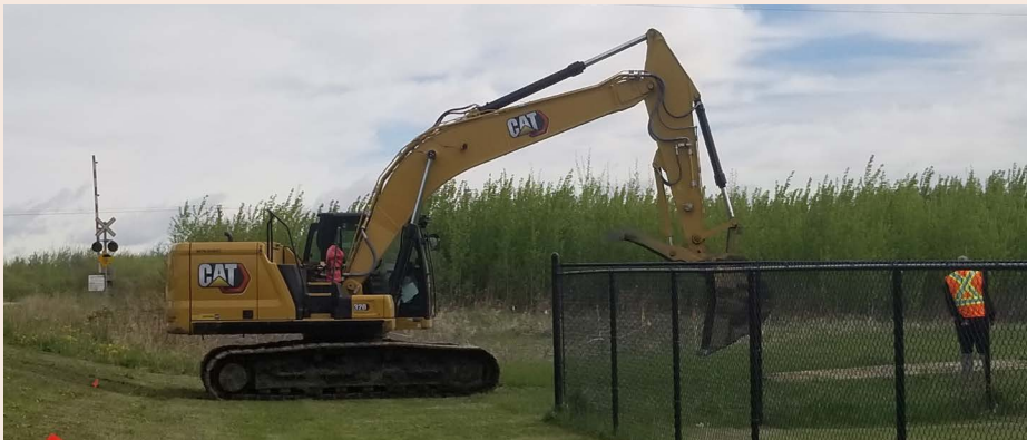
Dechant Construction Site preparation at Paul's Elementary Jr. High School
